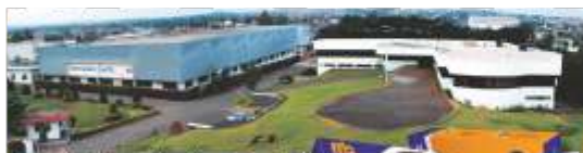
Menon Bearings plant at Kolhapur,
