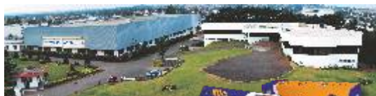
Menon Bearings plant at Kolhapur,
